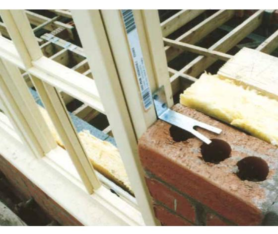
100 per box. Ties timber frames to masonry.
